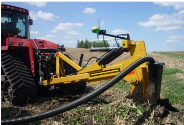
Drainage plow installing drain tubing in field.
